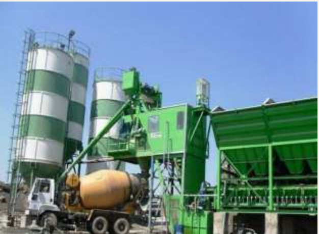
Ready Mix Concrete Plant on Site
